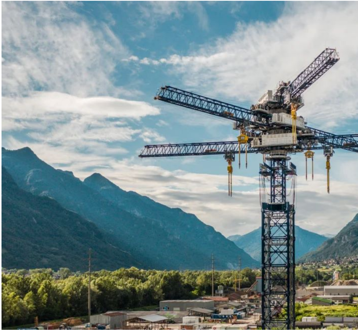
©Energy Vault Gravity storage
